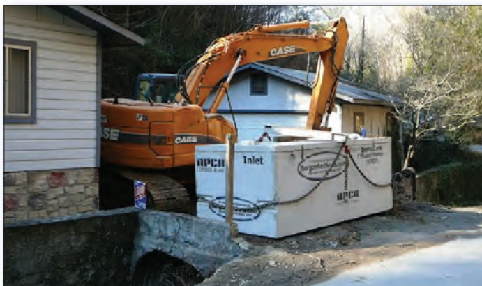
Figure 2. Maneuvering the new STEP system equipment into place was challenging because of tight working conditions along King Branch Road.
